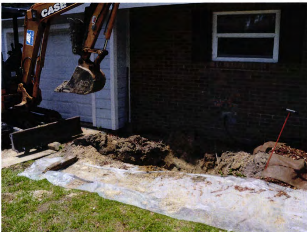
Picture 2: UST 1359 Cardinal excavation.
